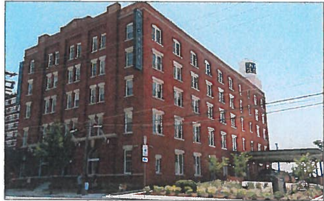
The 1910 building that once housed the Dallas Coffin Company has been rehabilitated into the Nylo Southside Boutique Hotel.
