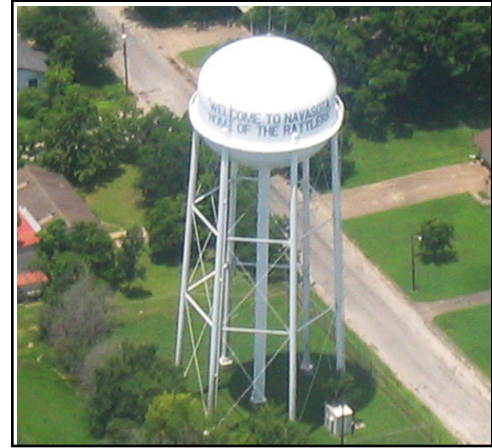
0.4 MG Elevated Water Tower
