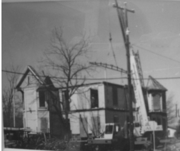
Two story house being dismantled for its trip to 951 S. Alamo
