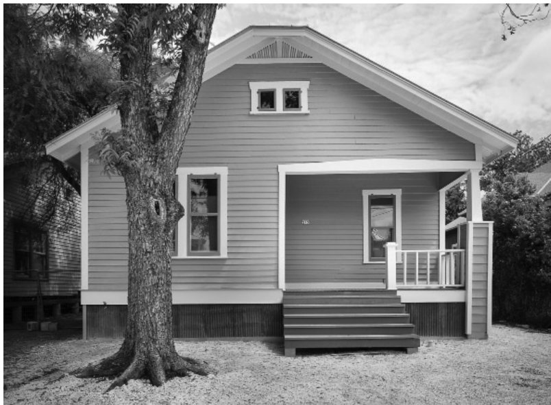
Street view of the Vance Street guest house showing storm windows configured like historic wooden screens. (Photo © Scott Martin)
