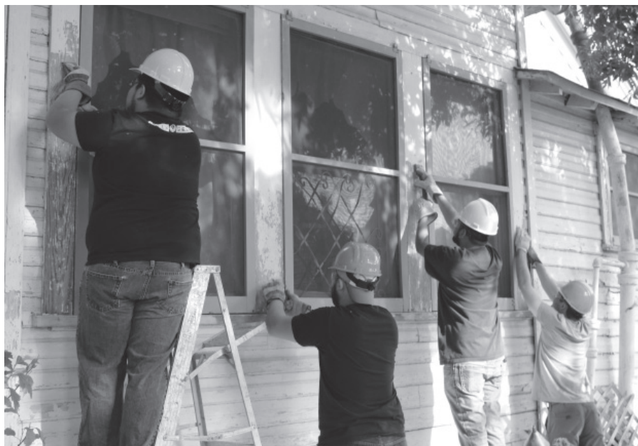
STAR volunteers work on Crofton St. house.
