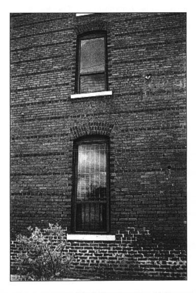
The upper portions of this brick masonry appear to be in good condition; however, the lower portions have lost mortar and have been poorly repointed.
