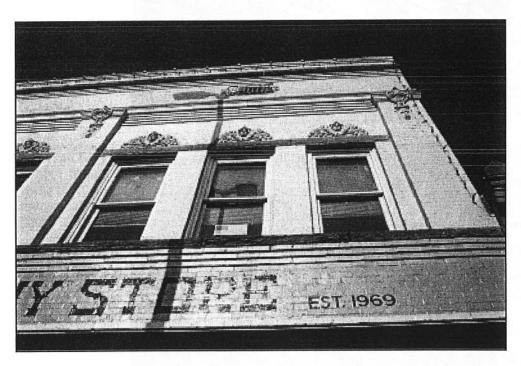
✓ The wood, double-hung windows in this building's second floor remain intact and provide light into the interior.
