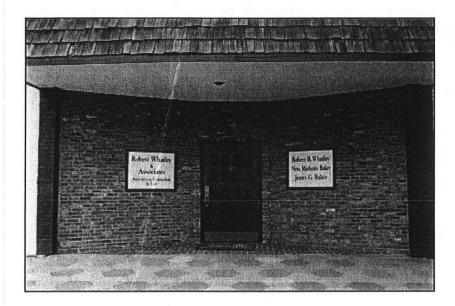
This building's originally open glass storefront has been completely infilled with solid materials.
