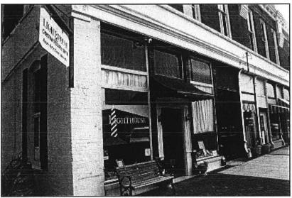
Cast-iron columns are used to support the weight of upper floors.
