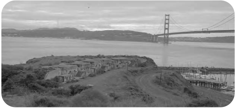
Battery George Yates, completed in 1905, is an excellent example of coastal fortification from the Endicott's period (1890 to 1905). Made of massive amounts of unreinforced concrete, this battery was constructed deep and low into the earth. Its stout construction and low-profile made it difficult for enemy gunfire to locate and attack. (photo circa 1973)
