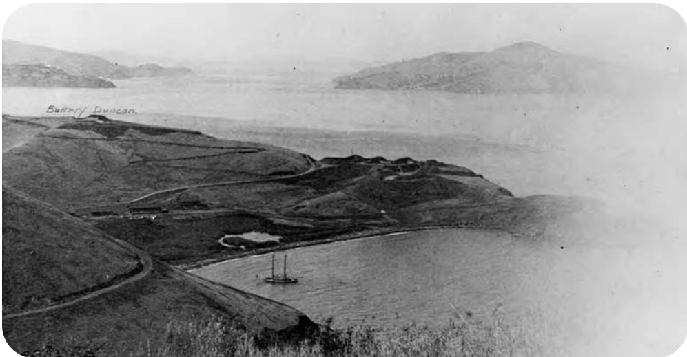
This early photo of Horseshoe Cove provides you with an idea of what this gentle harbor looked like around 1905. The military had already begun to shape the surrounding land with the construction of Batteries Cavallo, Yates and Duncan. But at the water's edge, before the buildings and the breakwaters were constructed, there was only a curving sand beach with brackish marsh land to the north. (photo circa 1905)
